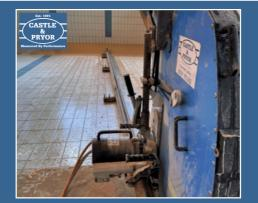
**TRACK SAWING** IN A SWIMMING POOL Cutting chases for pipes 14 metres long
